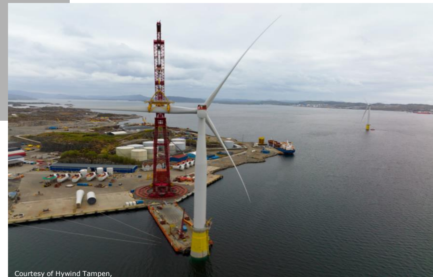
Courtesy of Hywind Tampen, https://www.offshorewind.biz/2022/05/23/first-turbines-assembled-for-hywind-tampen-floating-offshore-wind-farm/
