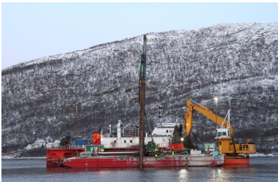
Picture 2. Positioning of pile - Kvalsundet (photo: NCA).
